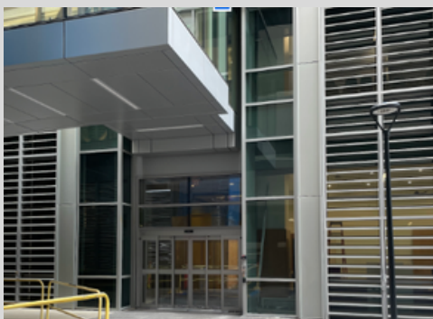
ENTRANCE FROM PARKING
